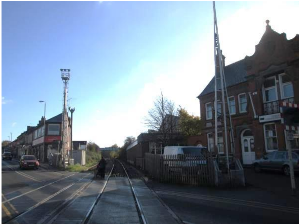
Image 8: Rail Crossing between Hotel Street and High Street
